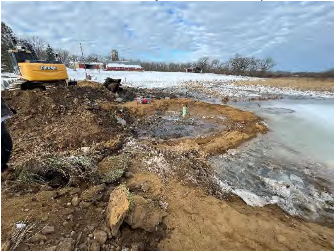
Earthen Dam to hold back water for culvert installation
