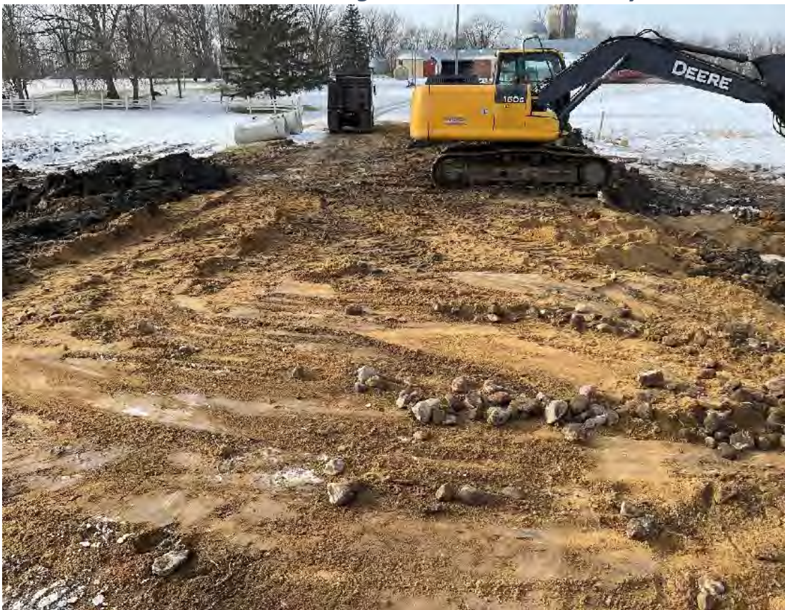
New Culverts installed and backfilled
