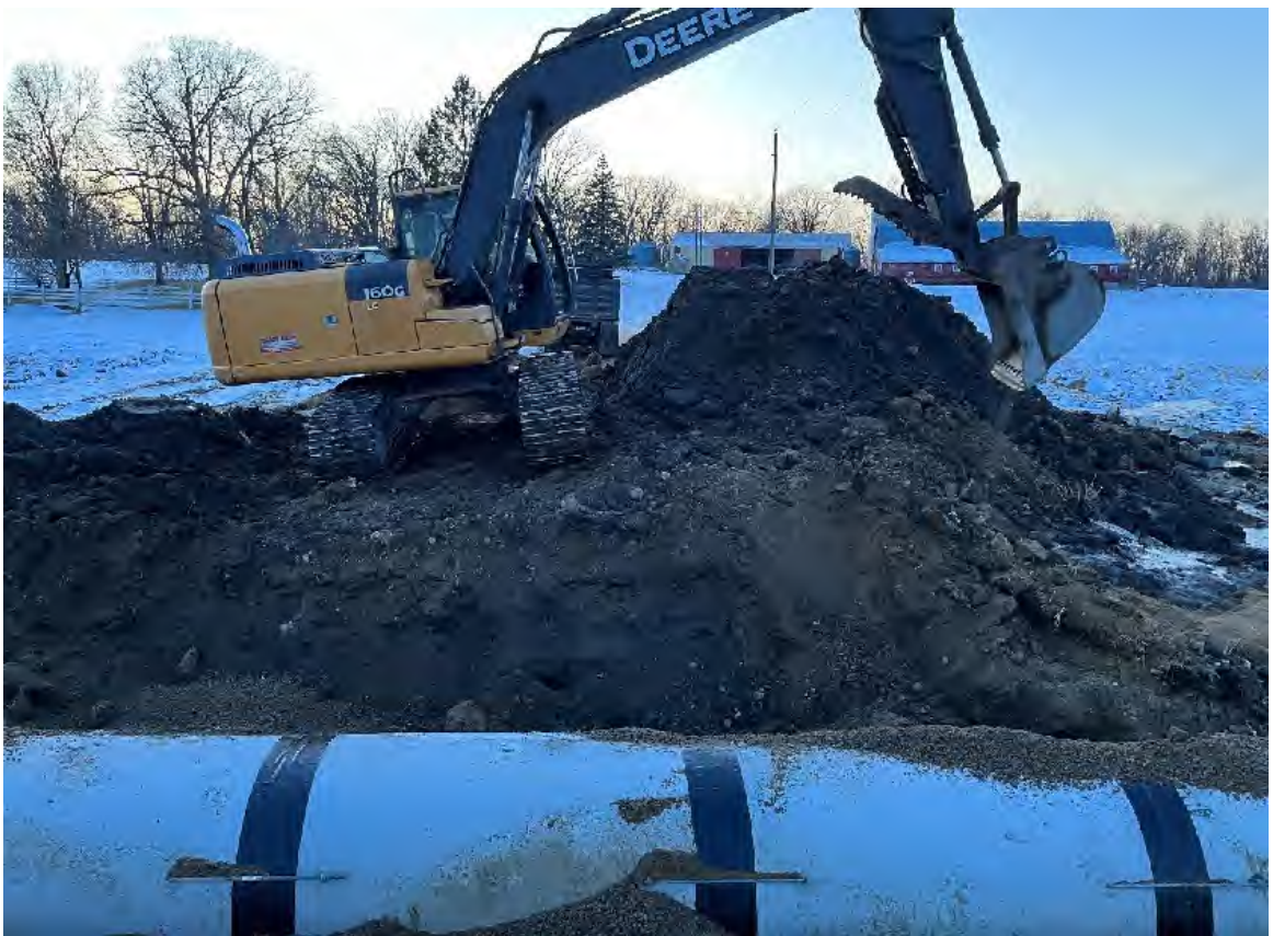
Contractor installing new culvert in driveway
