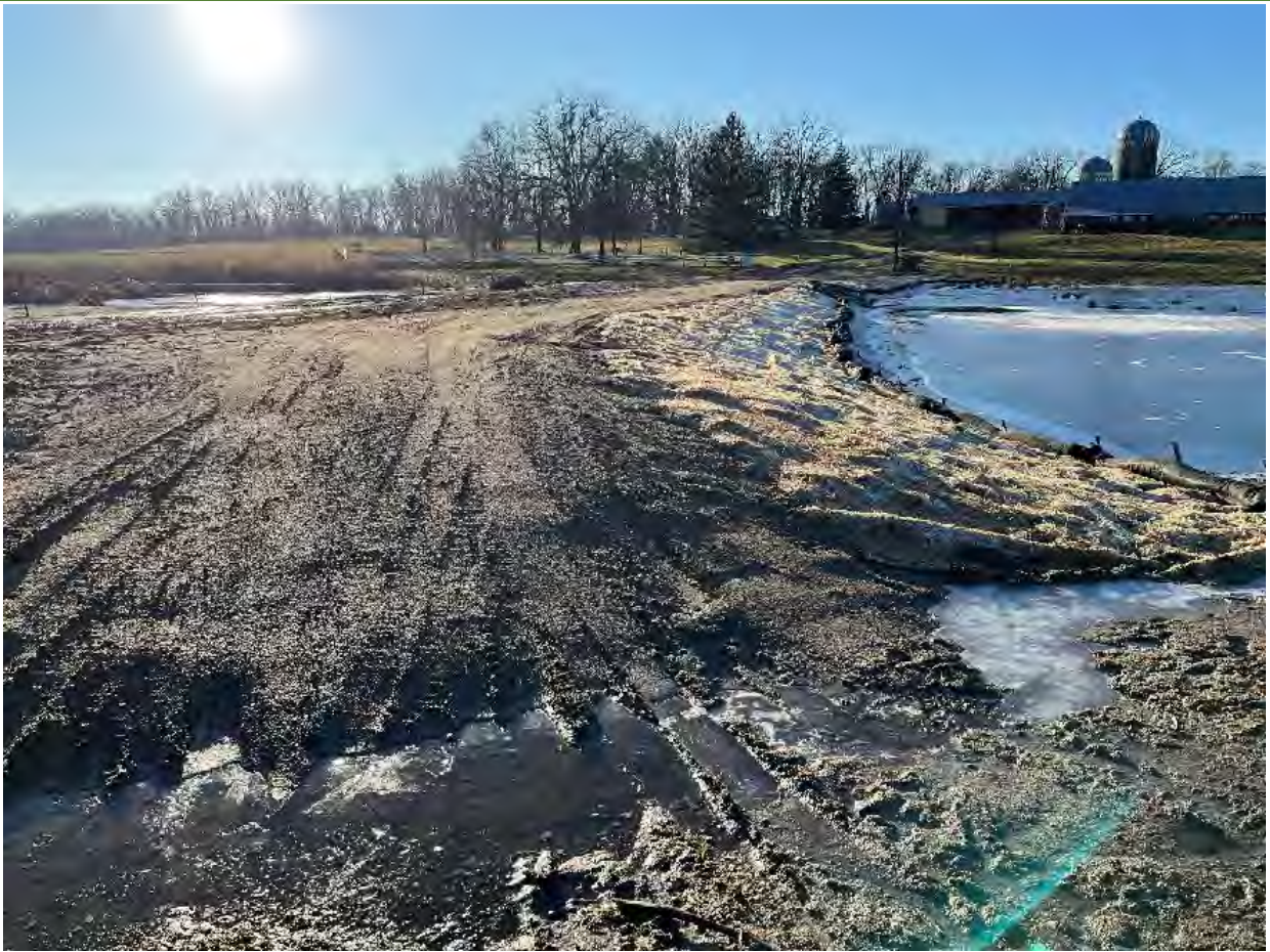
Completed Crossing with Erosion/Sediment Control BMPs in Place
