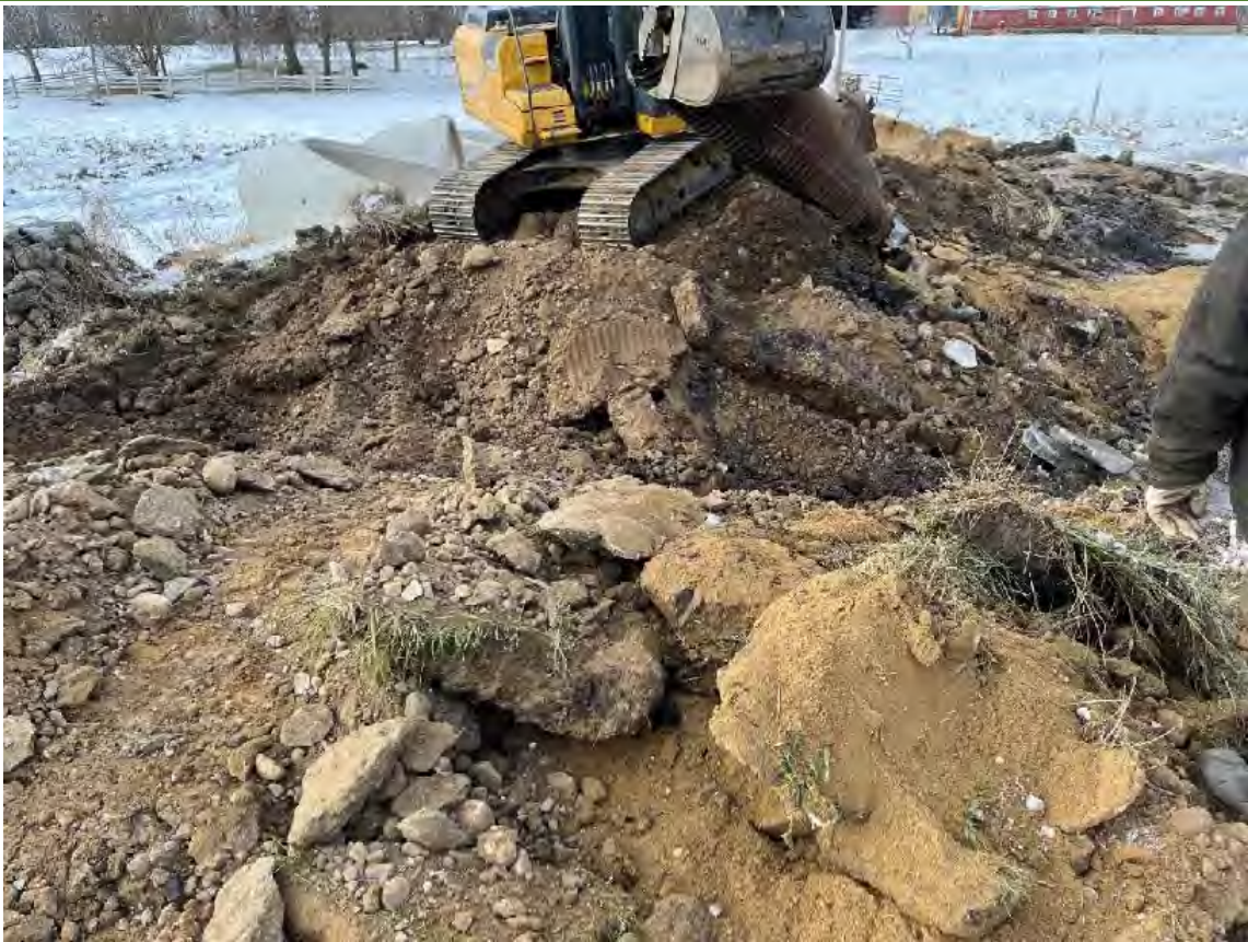
Contractor removing old culvert in driveway
